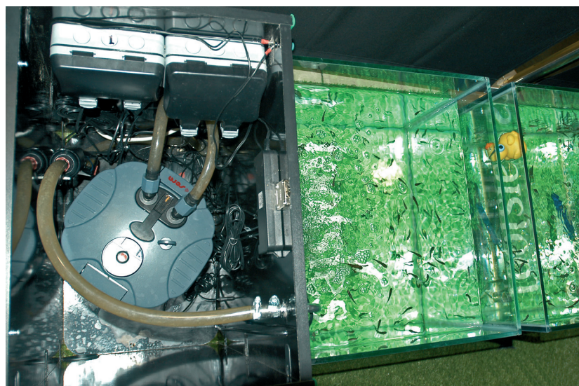
FIG 3: The external canister filtration and ultra-violet system is housed under the seating area.
