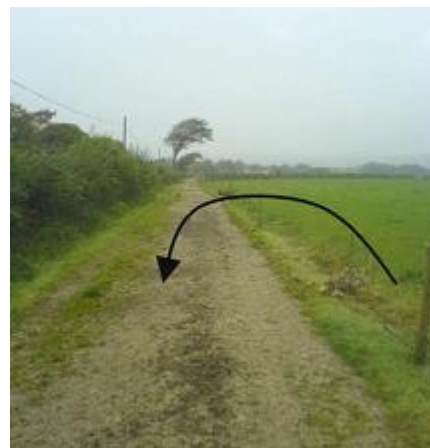
Fig 3: The 'up-and-over' involves digging up subsoil from next to the intended track, moving it over and onto the new track and back filling the topsoil
