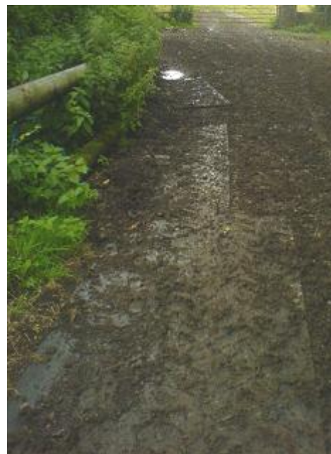
Fig 6: Quarry belting can be a portable solution
