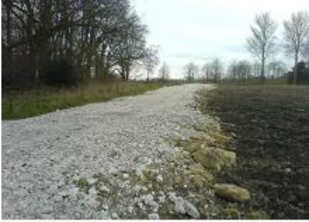
Fig 4: Investing effort in preparing a raised base will improve drainage. Some 'sinking' should be anticipated and an 'over-camber' is rarely the main concern.
