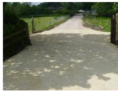
Fig 9: - Above is a picture of an oolitic limestone track. This material crushes to a fine material and self-stabilises. This can be achieved with hard stones and builders rubble (metal removed) by finely crushing, adding cement and compacting. Soft stone (limestone or sandstone) crumble rather than penetrate the white line. Similarly, pine peelings or wood chip prove very comfortable for cows, provided they are well drained. Achieving good drainage by raising the track, creating a camber to ditches and encouraging drying appears to be most important for lameness prevention. Other practical issues include regular maintenance including the removal of mud verges that form over time.
